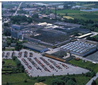
Stiebel Eltron's plant in Holzminden, Germany
